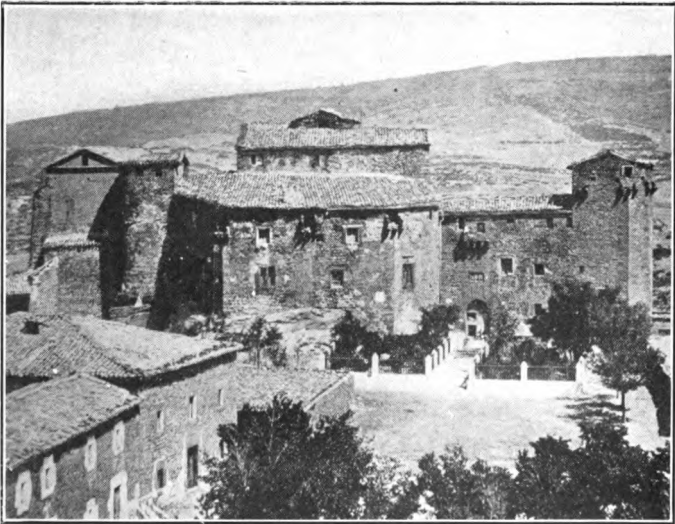
BIRTHPLACE OF ST. FRANCIS XAVIER (Before its Restoration)
